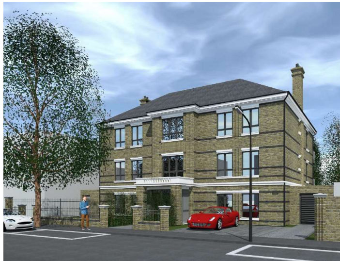
Figure 1 CGI of proposal (NOTE: minor changes have been made to the landscaping at the front)
